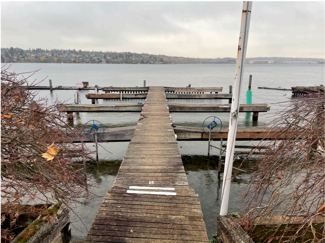
Photo 6 - D-dock looking waterward.
