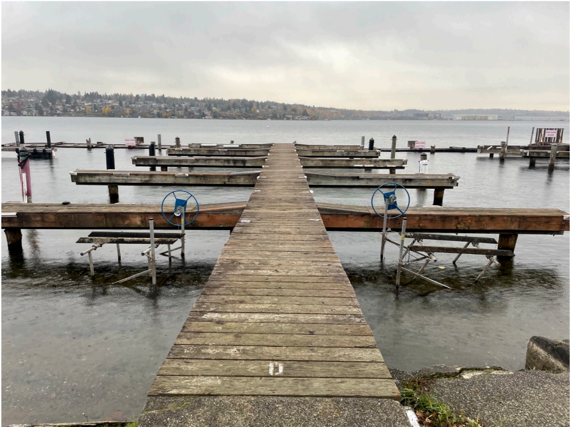
Photo 4 - B-dock looking waterward.
