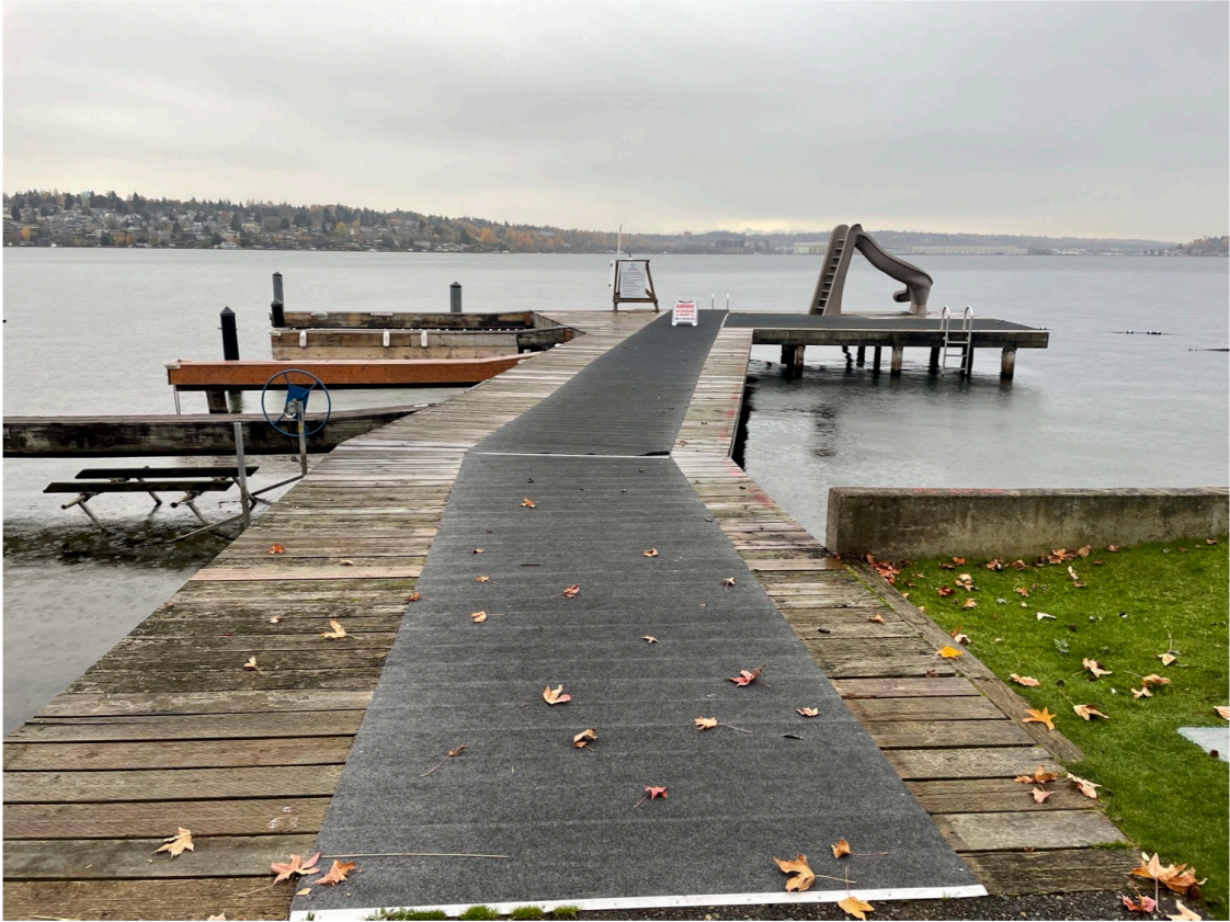
Photo 3 - Existing swim dock looking waterward.
