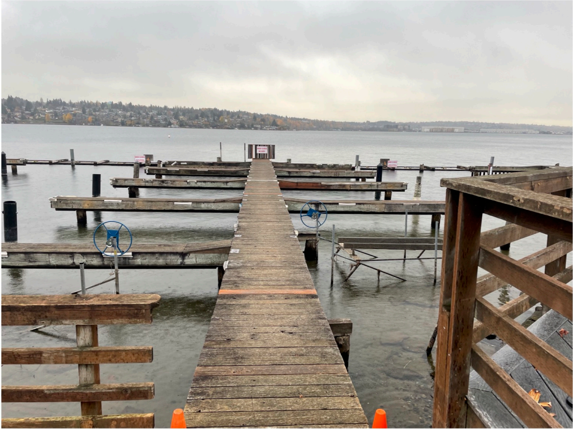
Photo 5 - C-dock looking waterward.
